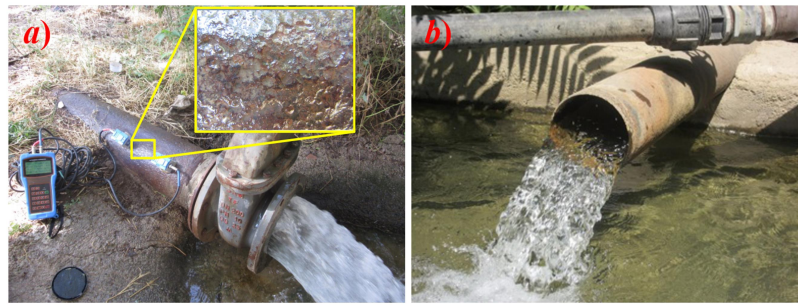
Figure 1. Well pump outlet: (a) Full pipe flow, (b) Partially filled pipe flow (photos by Mohammad Bijankhan, Alborz Province, Iran).
