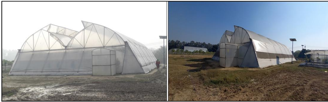
Figure 1. Front view of 560 m 2 polyhouse at PAU, Ludhiana.
