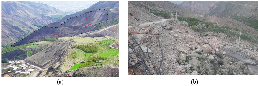
Figure 3. Two landslides that occurred and their damages: (a) South of Yaroud and (b) South of Viar Villages.
