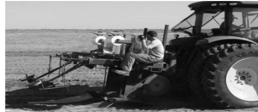
Figure 1. SWRT membrane installation equipment (Smucker and Basso, 2014).
